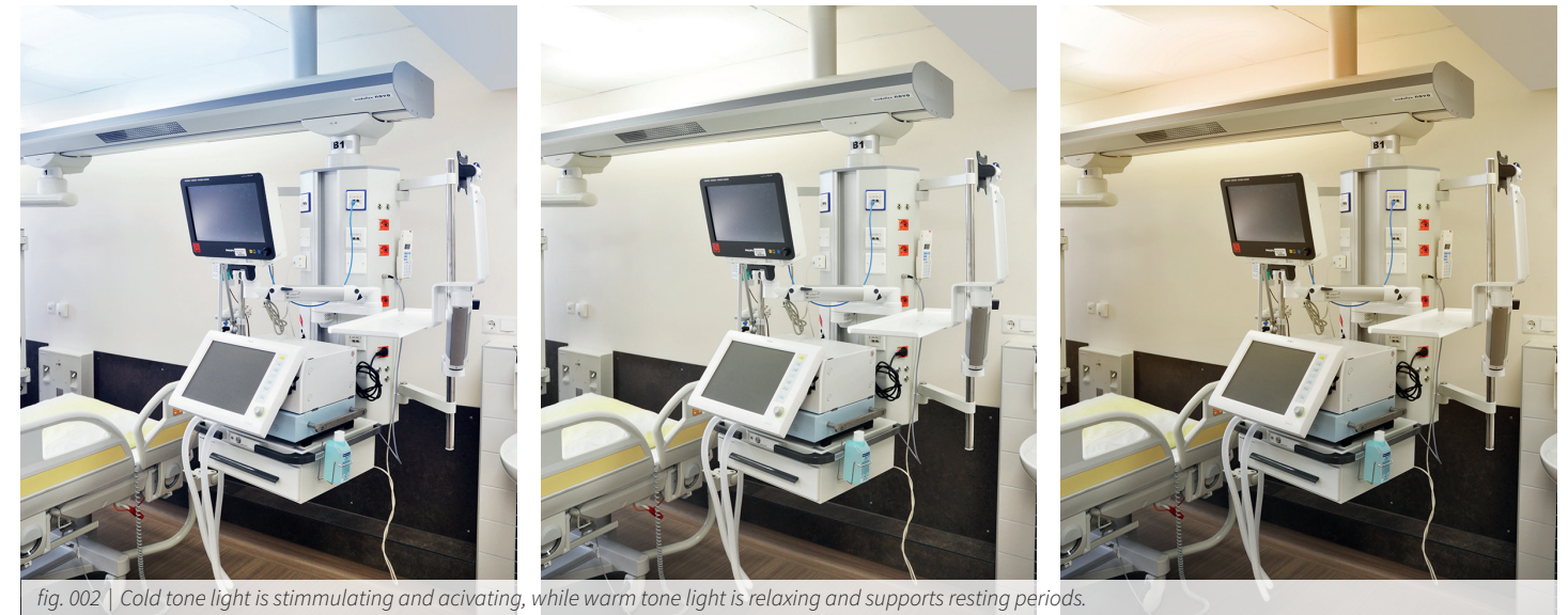
fig. 002 | Cold tone light is stimulating and activating, while warm tone light is relaxing and supports resting periods.
